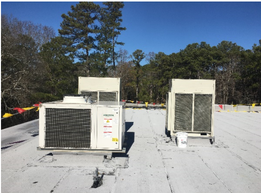
Relocated RTU Units
