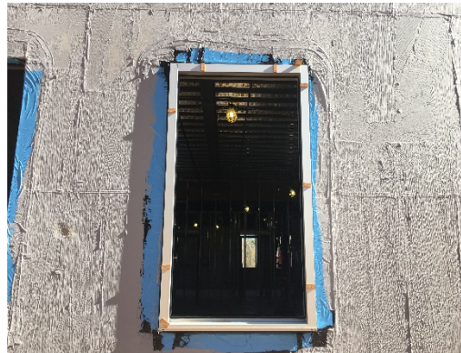
New Addition Window Framing & AWB
