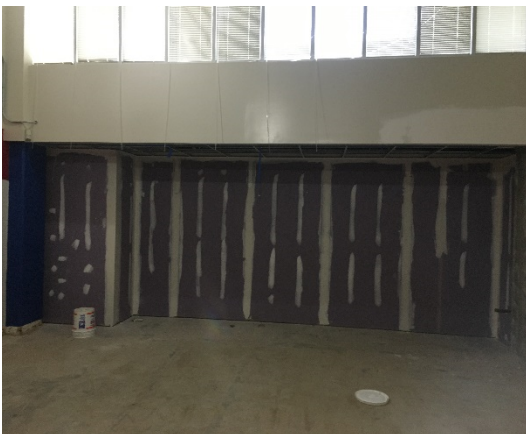
Building #2032 Drywall Tape & Finish
