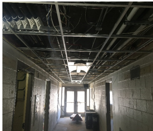
Building #2032 Ceiling Grid Installation
