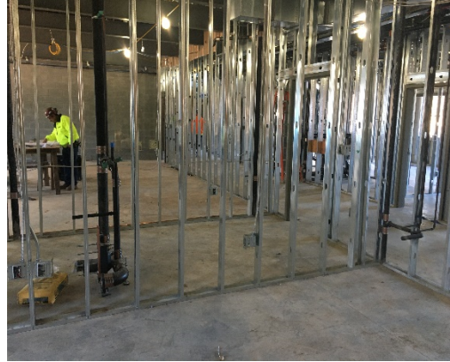
New Addition In Wall MEP
